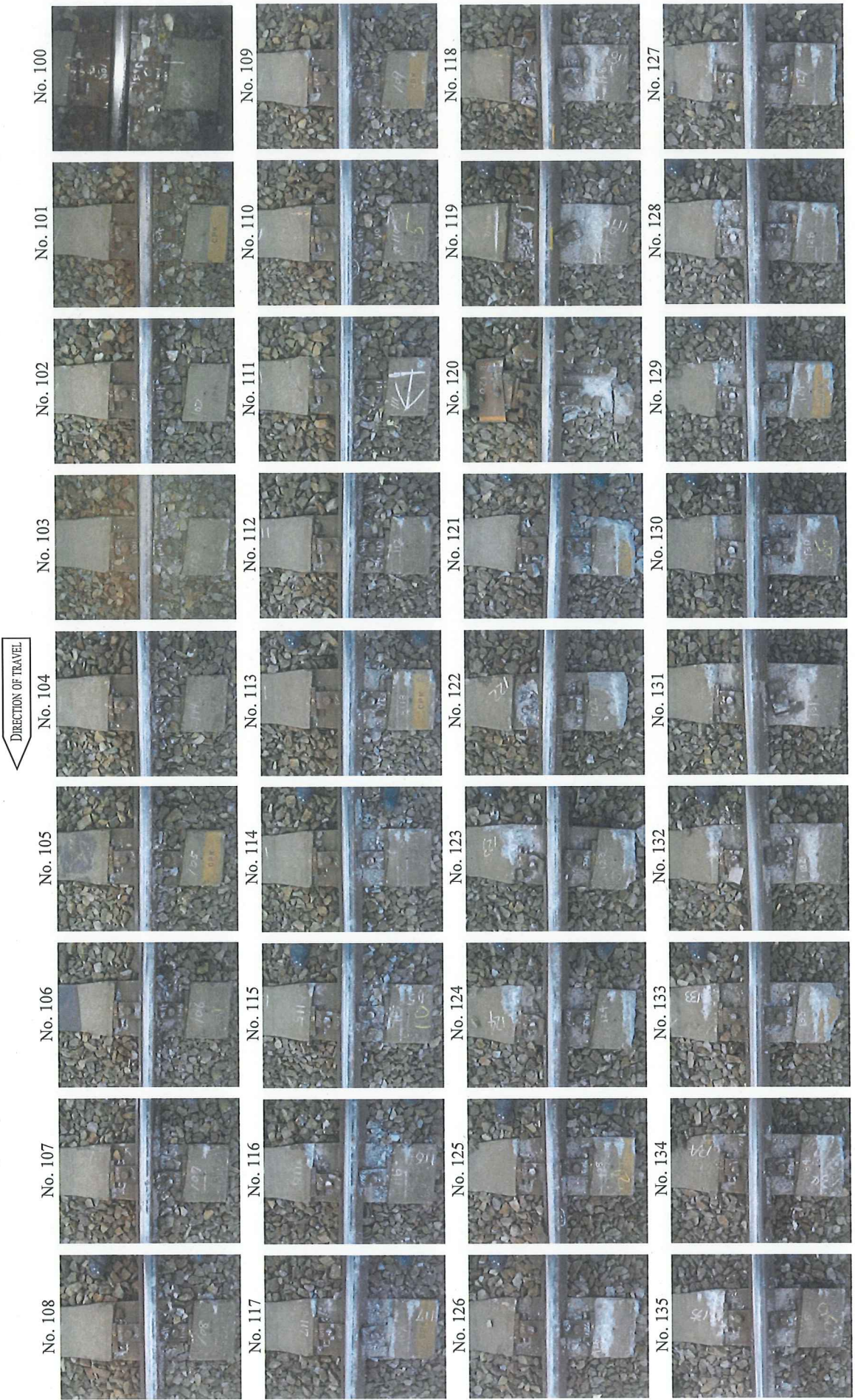
Figure 7 - States of Damage to Railway Facilities etc. (4) (Sleepers on the left rail side of the up track, 1/3)
