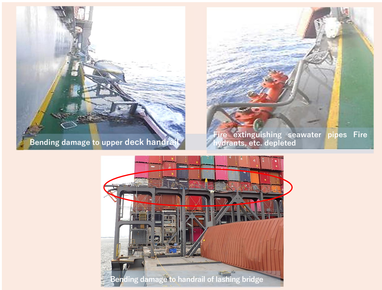
Photo 3 Damage to equipment on deck
