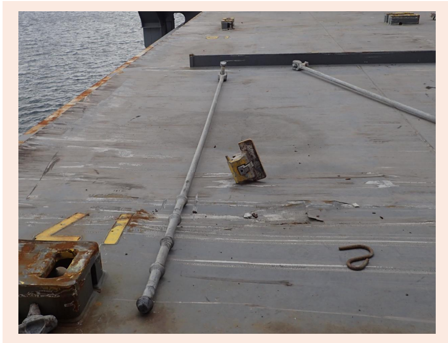
Photo 1 Container hatch cover
