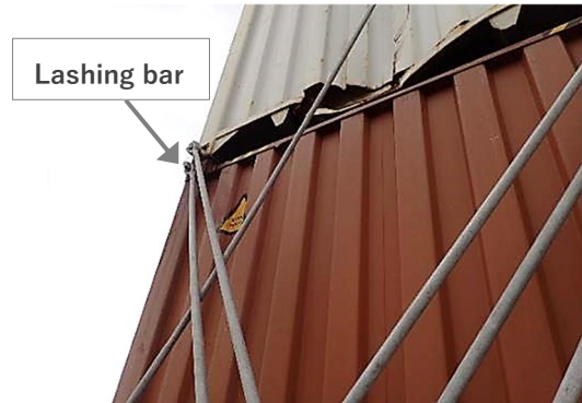
Photo 18: Lashing bar condition
