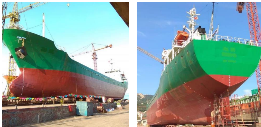
Photo 1 The Vessel (before the accident)
