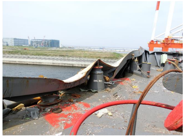
Damaged recessed bulwark
