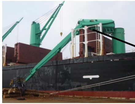
Photograph 3: The collapse of the crane
