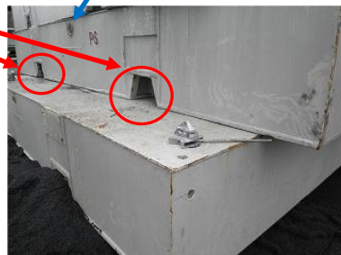
Photo 2.6-5 Side surface of tween deck hatch cover
