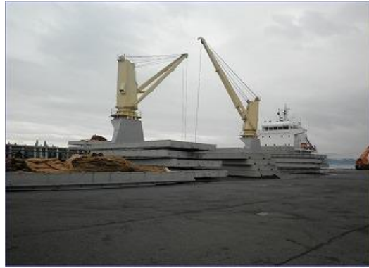
Photo 2.1-12 The Ship, and upper deck hatch covers that were moved to the wharf
