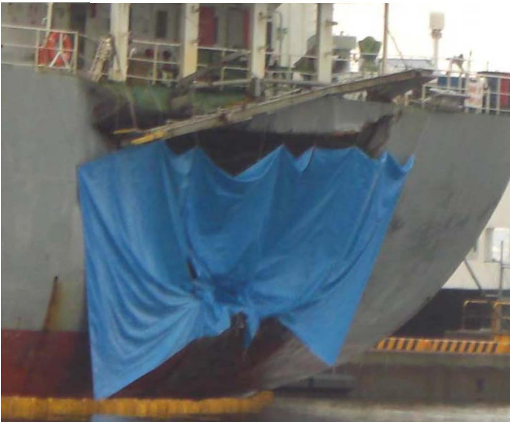
Photo 2: Damage to Ship A (Port Stern)
