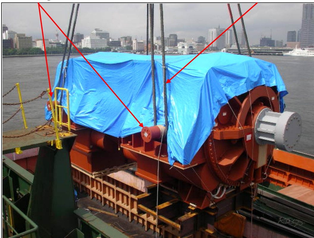
Loading Operation (immediately before the accident)
