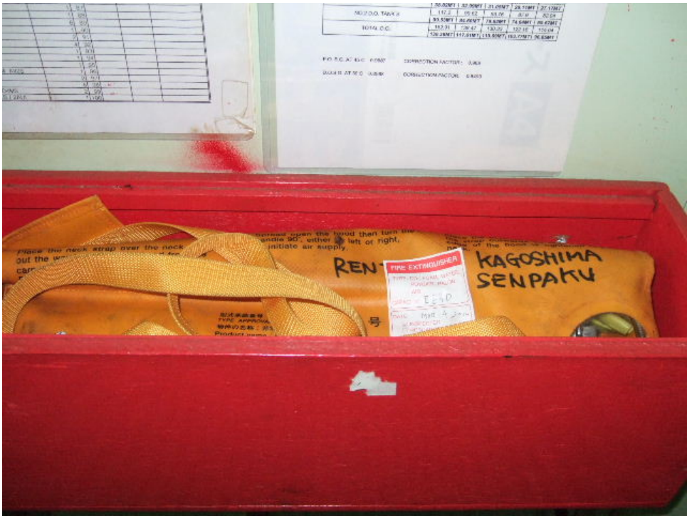
Photo 13: EEBD (Engine Control Room)
