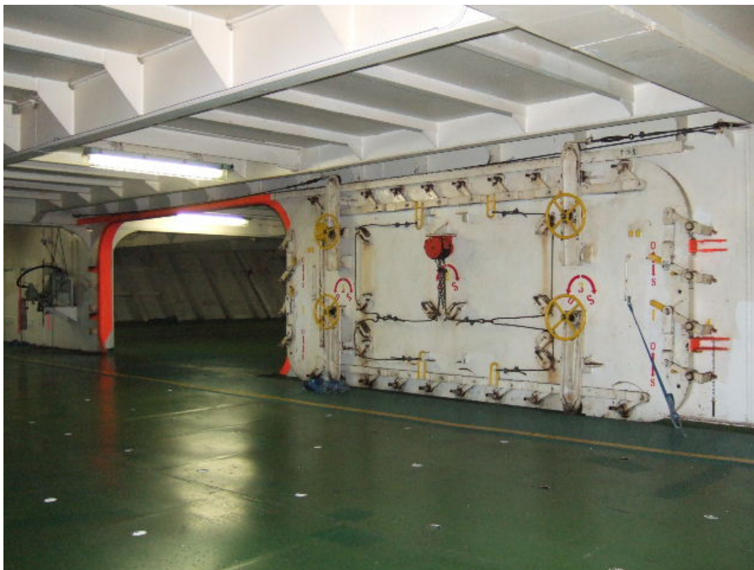
Photo 6: Sliding Bulkhead Door
