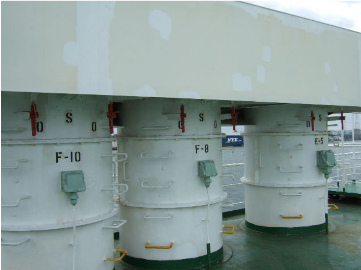
Photo 9: Ventilator (Dampers and Ventilation Holes)
