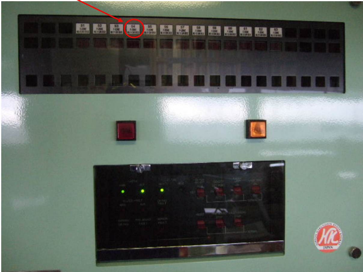
Photo 10: Smoke Detector Control Panel
