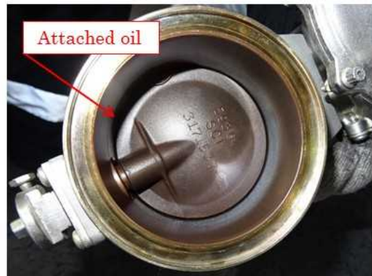
PRSOV(at side of No.2 Engine)
