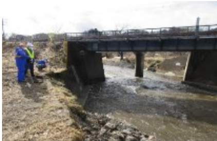
Figure 22: Completion of work (Full view)
