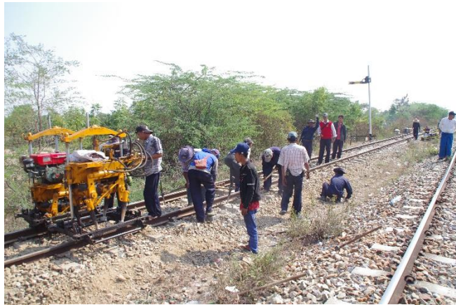
Work on track maintenance
