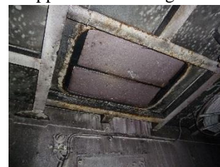
Welded Escape Hatch on Upper Deck Ceiling
